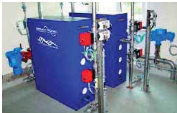
Results of ultrasound HPUS units installed at the Bamberg water resource recovery facility. Photo by Ultrawaves
