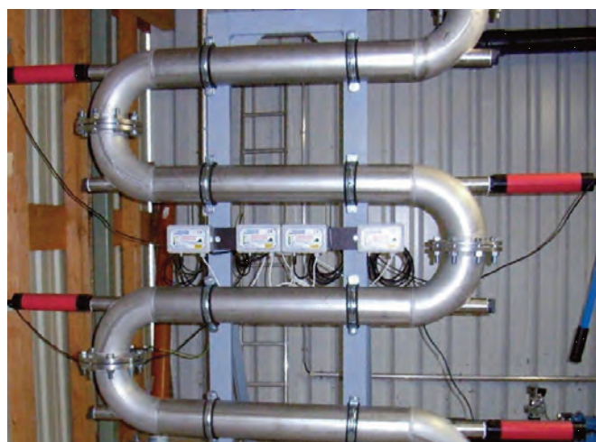
Fig. 2. Biocrack electrokinetical disintegration tube
