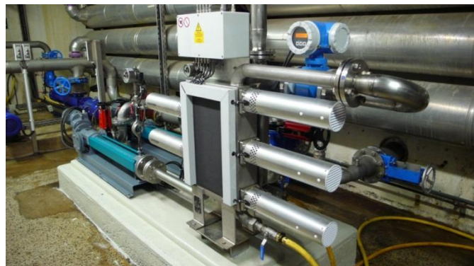
Figure 1: Integration of the ultrasound system (US)
