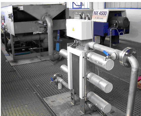
Figure 1: Scheme of sludge treatment on WWTP Bünde and Ultrasound system with thickener
